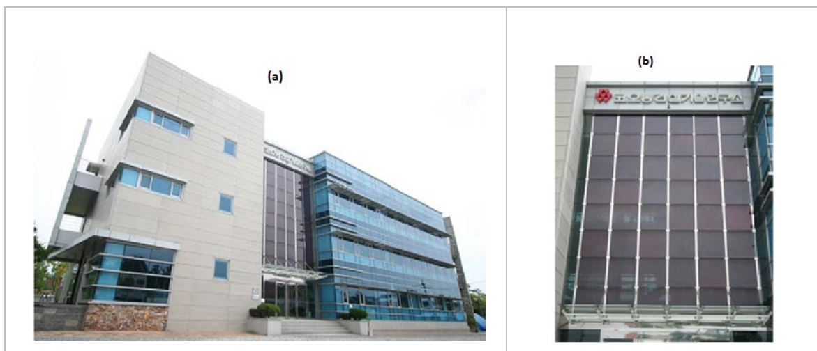
Figure 5: Application of thin-film Photovoltaic modules in institution building, (a) building front view, (b) part of the building having Photovoltaic modules [Yoon et al., 2013].
